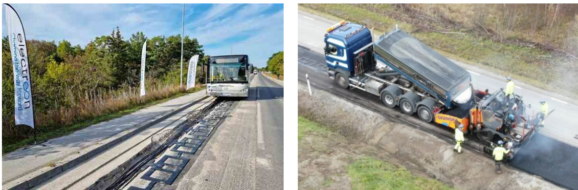
Figure 1 – Placement of inductive charging coils in a trench and asphalt paving for inductive pavement construction (Smartroad Gotland, 2022)
