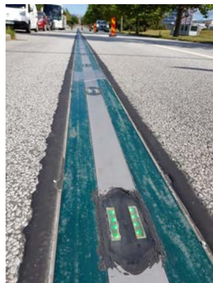
Figure 1 Conductive rail installed on a road
