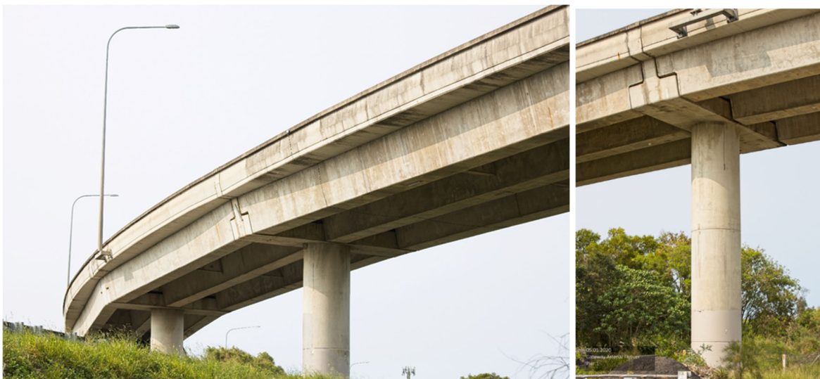
Figure 8 Halving joints on cantilever piers supporting Gateway Arterial Flyover (GAF)
