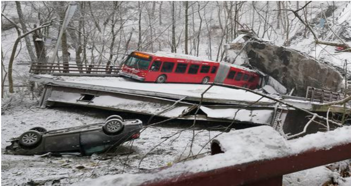
Figure 1 – Pittsburgh Bridge collapse on 28th January 2022 – see below:
