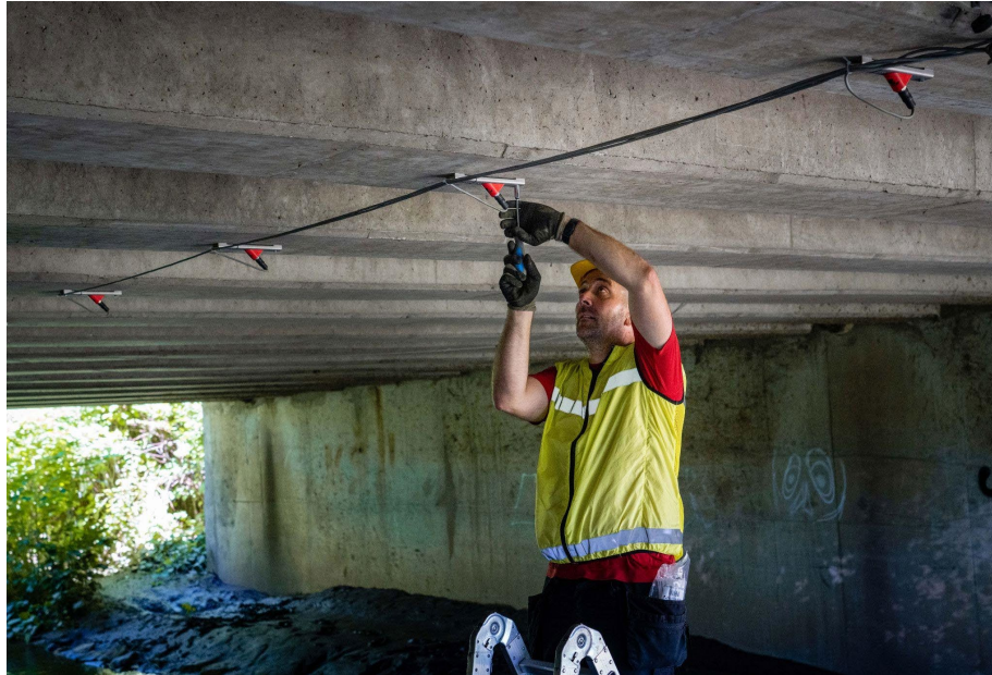
Figure 3 – Installation of bridge WIM sensors
