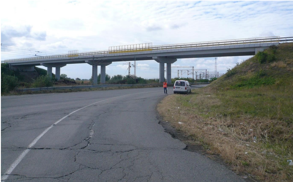
Figure 4 – Location of the installation of the bridge WIM system
