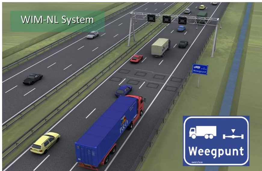
Figure 1 – WIM system consisting of a combination of in-road sensors and video images
