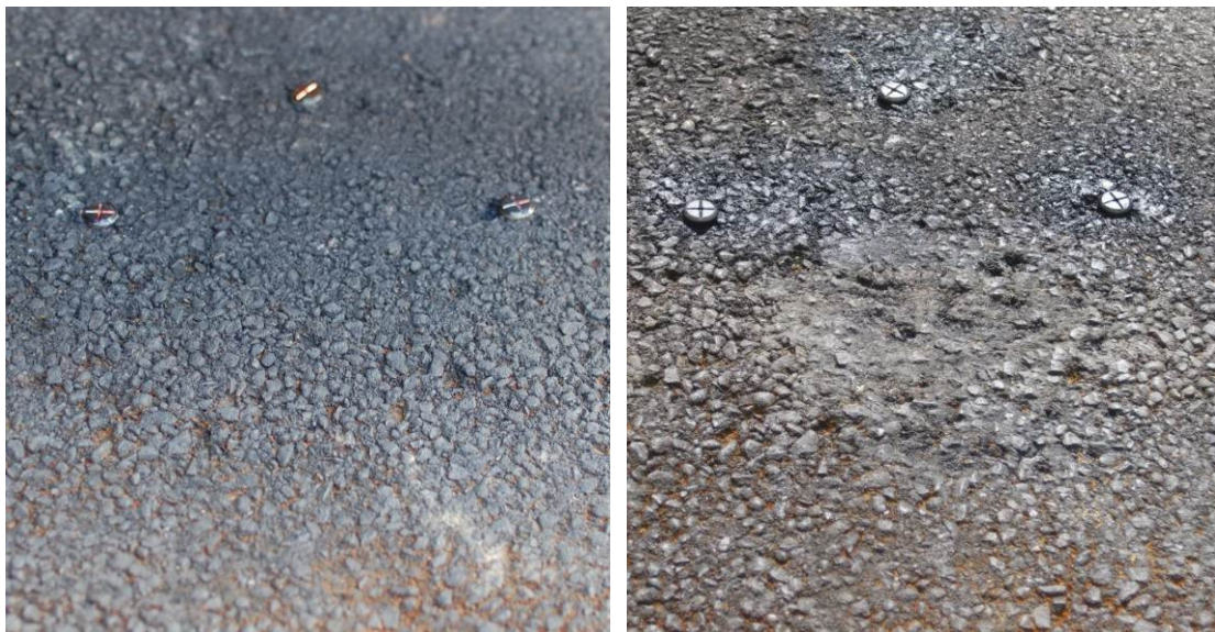
Figure 4 – Lightly-trafficked (left) and post-wear (right) hot mix asphalt surface
